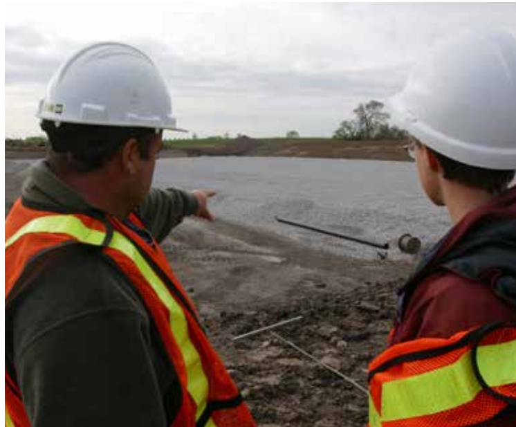
Construction of leachate collection system in Phase 2 prior to placement of garbage
