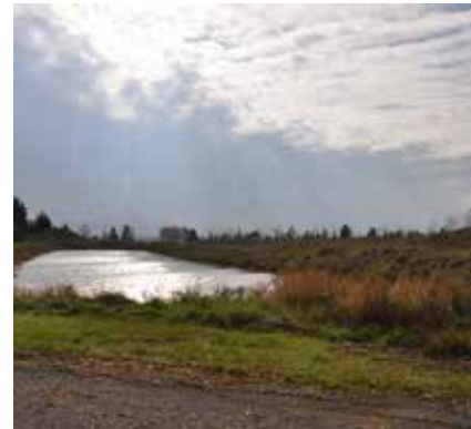
Forebay for existing Stormwater Management Pond
