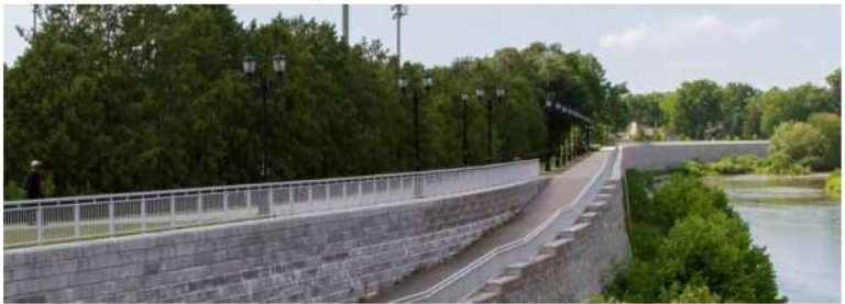
Existing West London Dyke, north of Kensington Bridge Source: City of London Get Involved webpage
