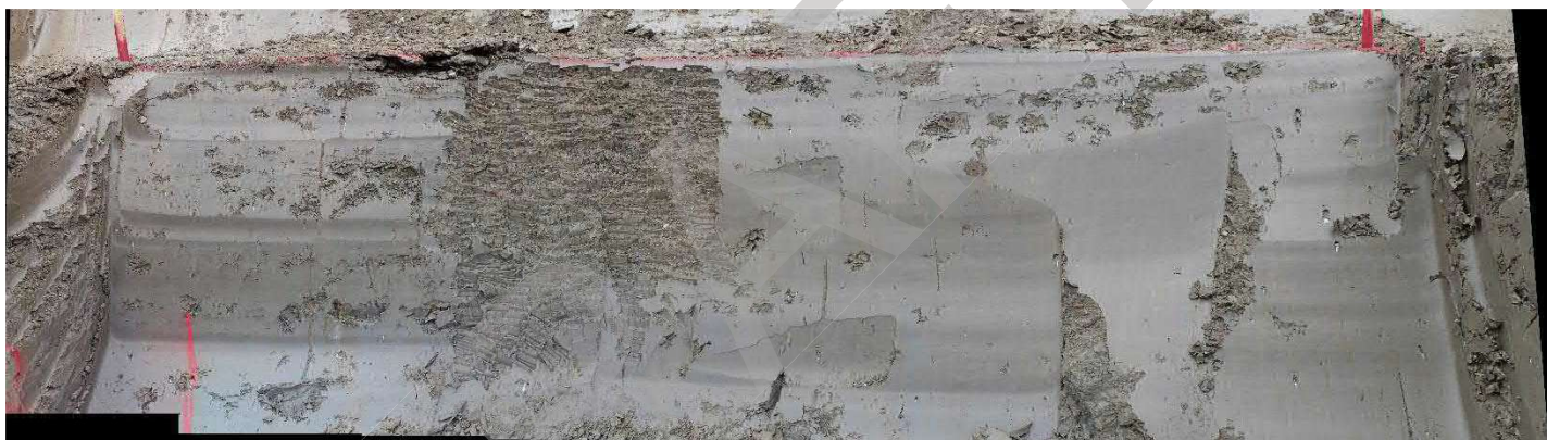
Photograph 16 Bench 3, facing north
