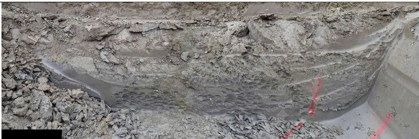
Photograph 15 Bench 3, facing west
