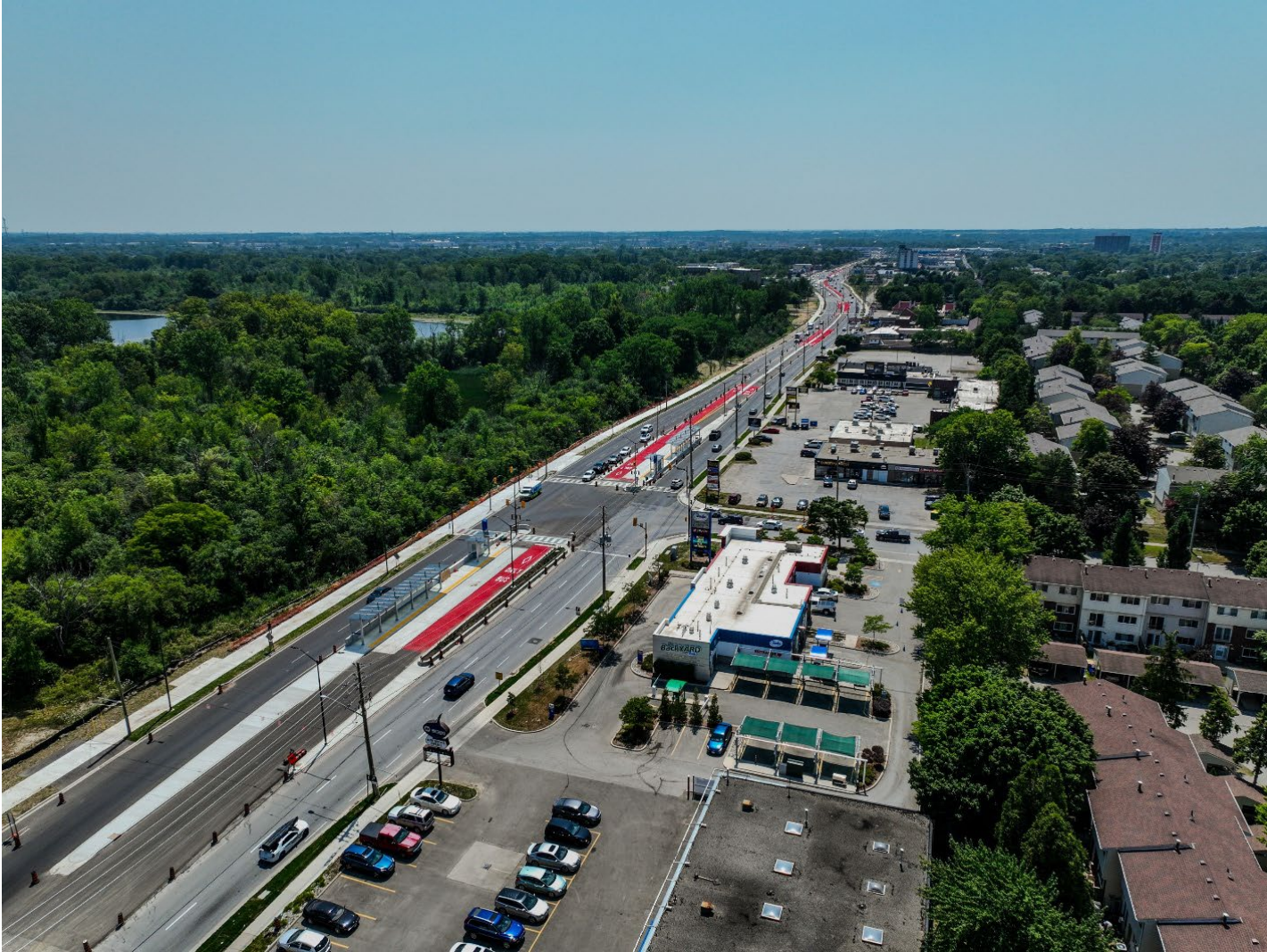
Aerial of Wellington Gateway Phase 3 looking south from Wilkins street (Complete with clean-up work ongoing until Fall 2026)
