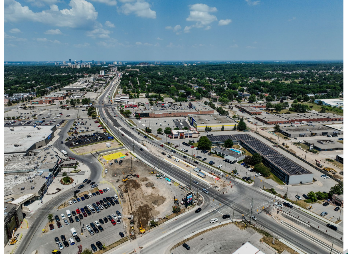
Aerial of Wellington Gateway Phase 4 at White Oaks Mall (Anticipated completion by the end of 2026)
