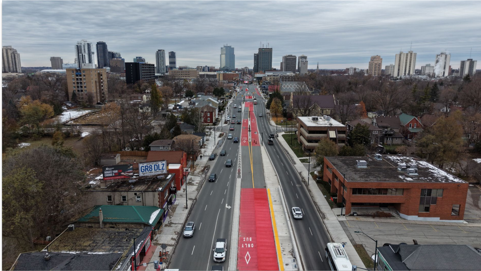
Wellington Gateway Phase 1 facing north from the Thames River (Completed in 2024)
