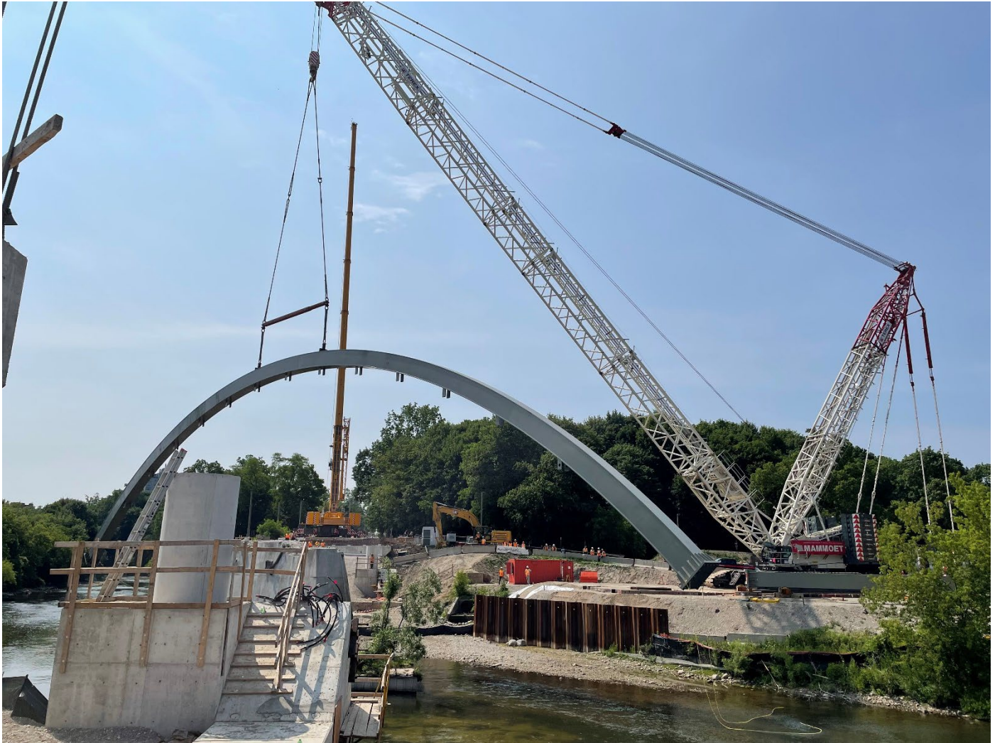
Above: The first of the two steel arches is lifted into place as part of the Victoria Bridge reconstruction project.
