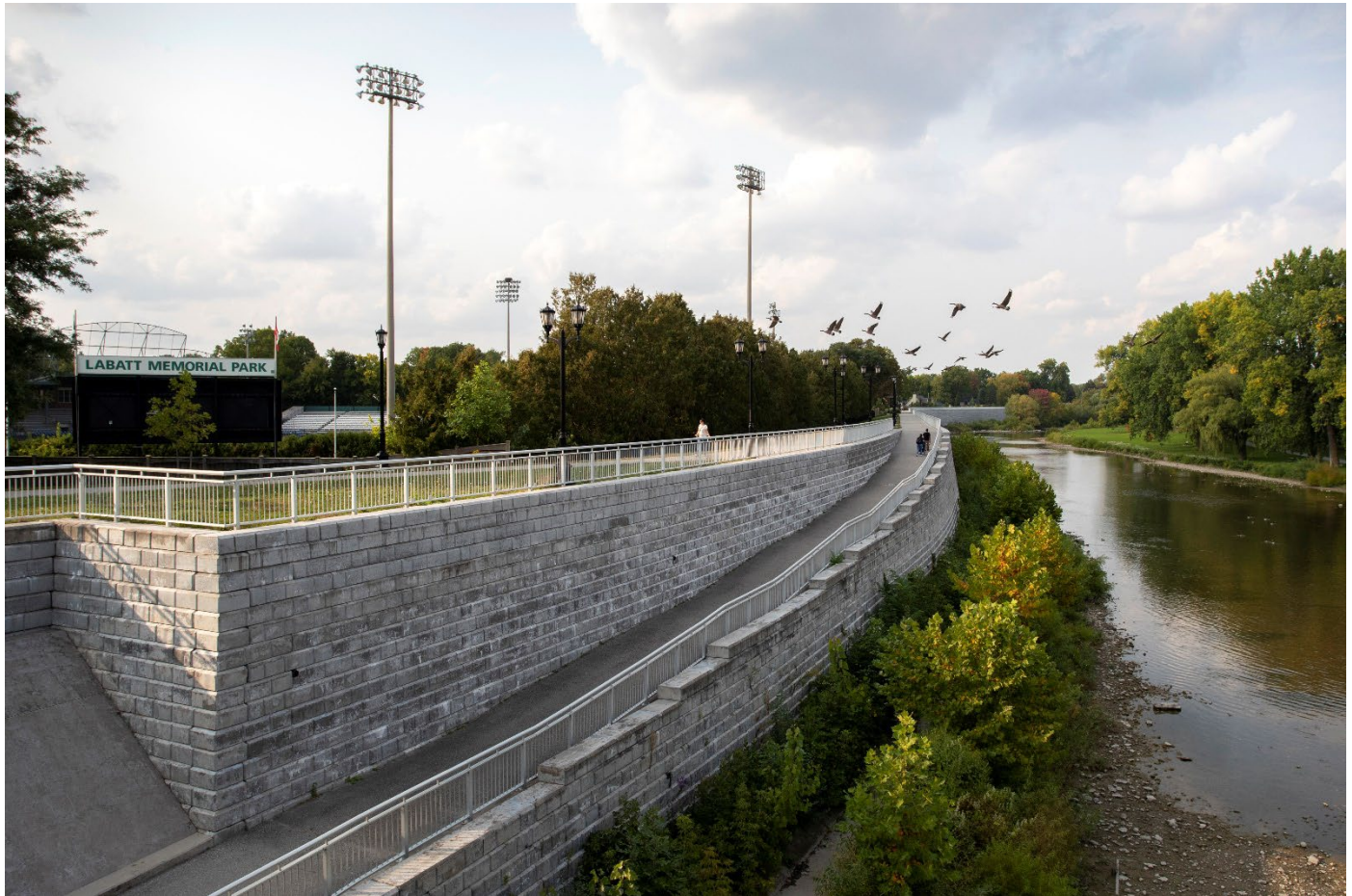
Above: The West London Dyke at the Forks of the Thames. Additional improvements are ongoing as part of the West London Dyke Master Repair Plan
