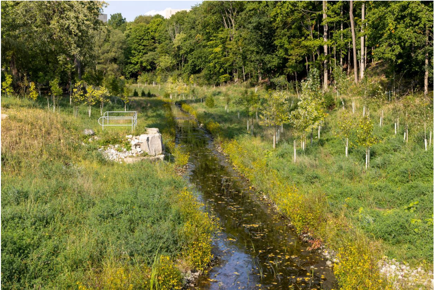
Above: The completed first phase of the Mud Creek rehabilitation project included a natural channel between CN Rail and Oxford Street.
