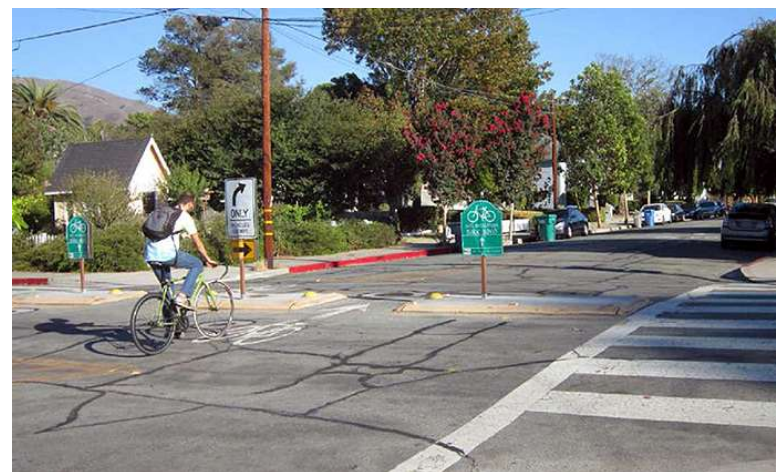
Intersection median island Source: Eugene Jud, Jud Consultants
