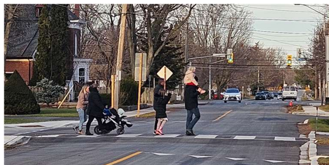
Raised Pedestrian Crossing
