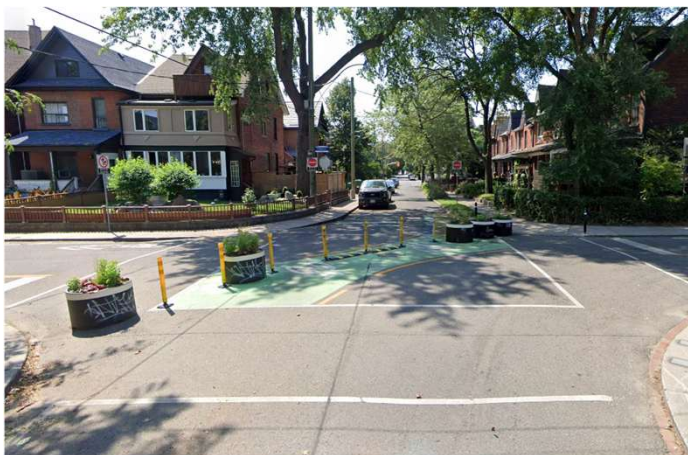
Temporary directional diverter at Lindsey Ave and Gladstone Ave
