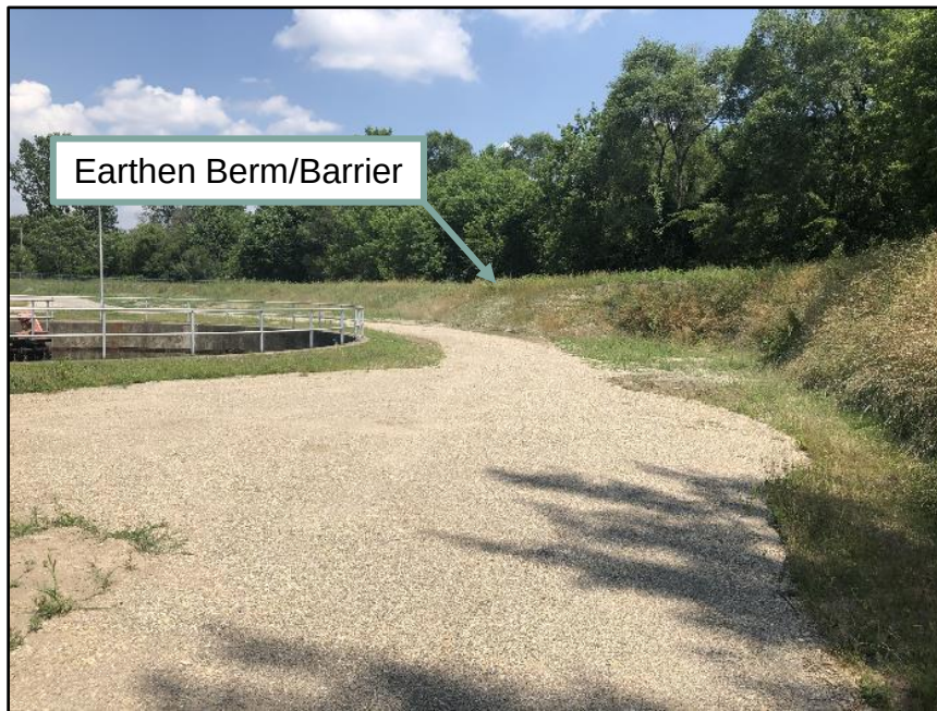
Earthen berm/barrier at the Vauxhall Wastewater Treatment Plant (City of London)
