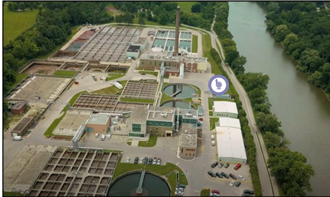
Proposed location of new Greenway WWTP Effluent Pump Station (Image Source: City of London)
