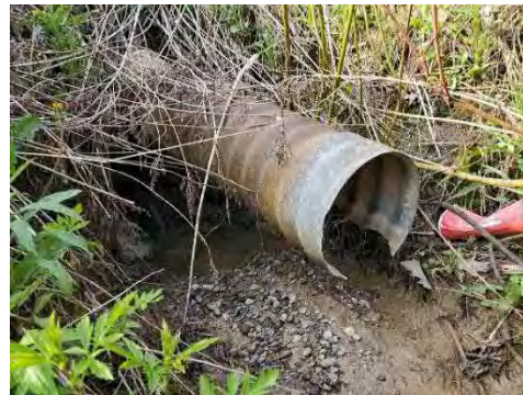
Photo 2: Location 1 – Culvert Outlet
