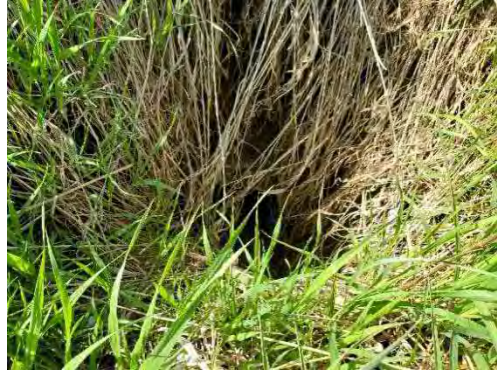
Photo 8: Location 3 – Culvert Outlet
