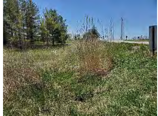
Photo 34: Location 12 – Culvert Outlet
