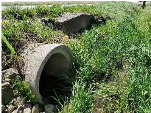
Photo 24: Location 9 – Culvert Inlet
