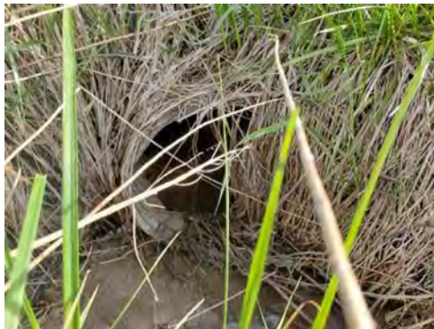
Photo 1: Location 1 – Culvert Inlet
