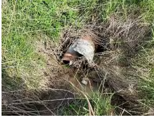
Photo 3: Location 2 – Culvert Inlet
