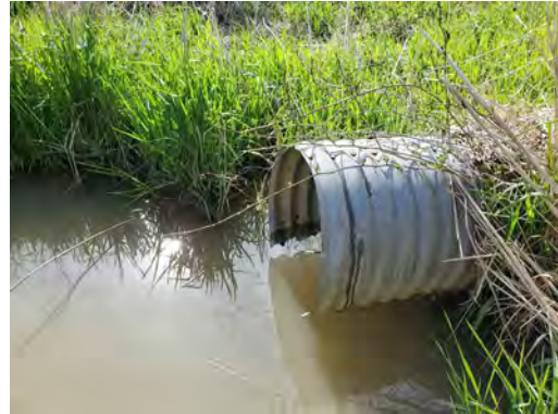
Photo 13: Location 5 – Culvert Outlet
