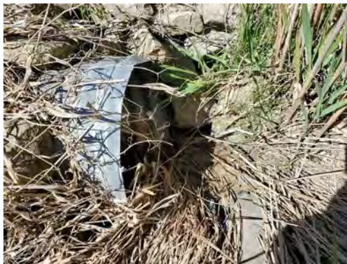
Photo 38: Location 14 – Culvert Inlet
