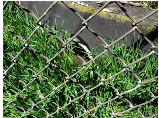
Photo 23: Location 9 – Pipe Outlet Upstream of Culvert
