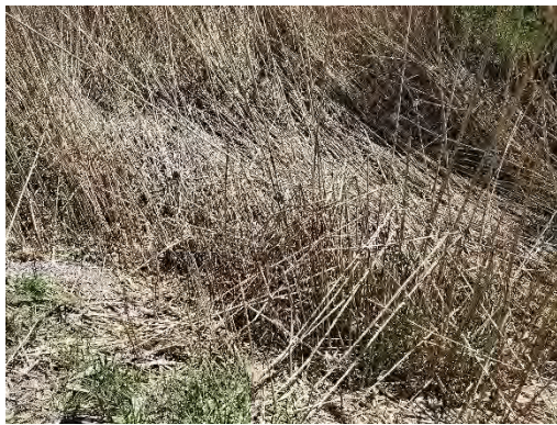
Photo 32: Location 11 – Culvert Outlet
