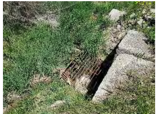
Photo 25: Location 9 – Grate Inlet near Culvert
