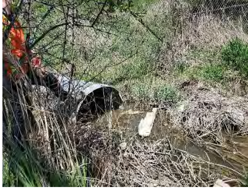
Photo 27: Location 10 – Outlet Pipe from Landfill
