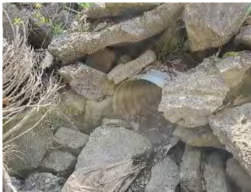
Photo 4: Location 2 – Culvert Outlet
