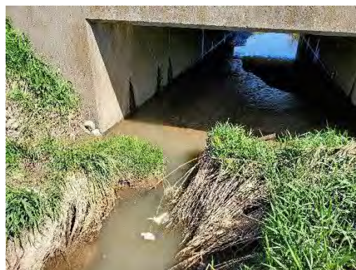
Photo 19: Location 8 – Box Culvert Downstream
