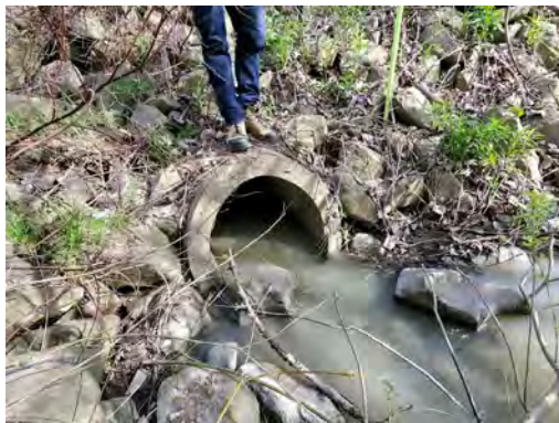
Photo 16: Location 7 – Culvert Inlet
