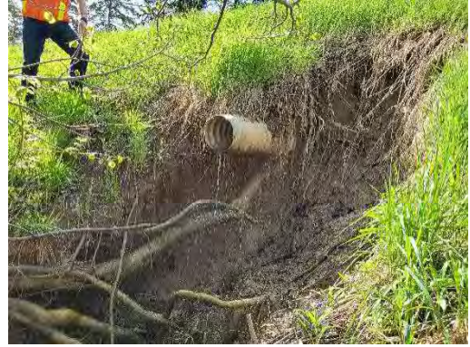
Photo 15: Location 6 – Culvert Outlet
