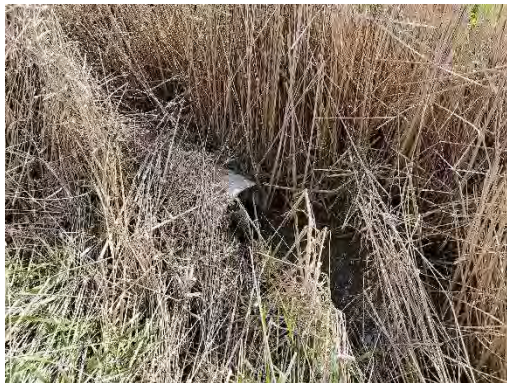
Photo 12: Location 5 – Culvert Inlet
