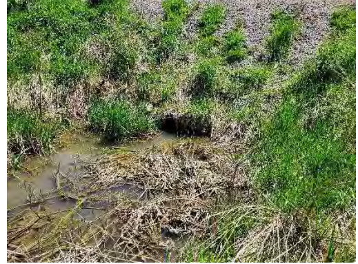
Photo 28: Location 10 – Culvert Inlet
