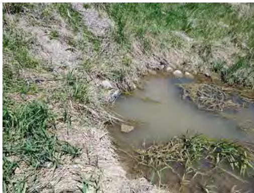
Photo 29: Location 10 – Culvert Outlet
