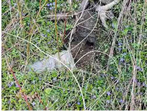
Photo 14: Location 6 – Culvert Inlet
