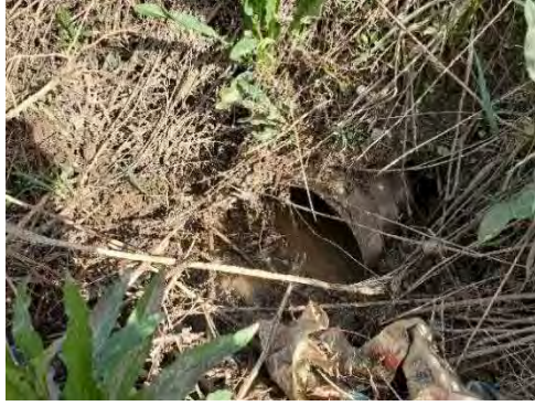
Photo 6: Location 3 – Culvert Inlet
