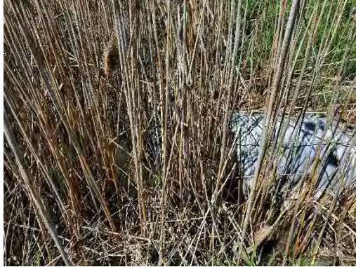
Photo 37: Location 13 – Culvert Outlet
