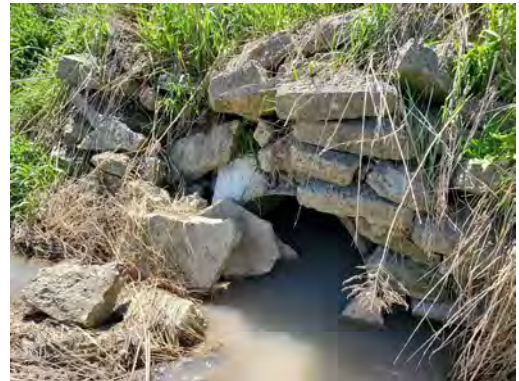
Photo 36: Location 13 – Culvert Inlet
