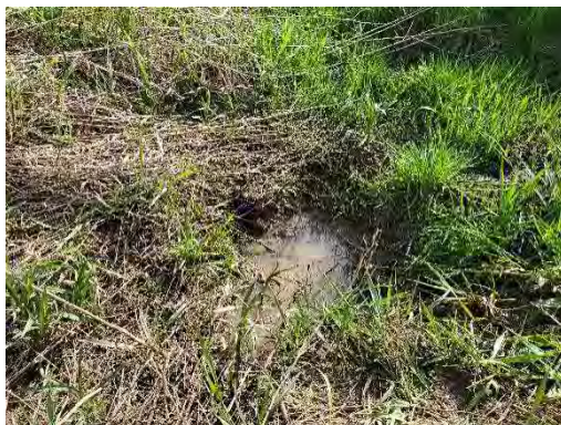
Photo 9: Location 4 – Culvert Inlet
