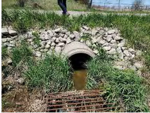
Photo 26: Location 9 – Culvert Outlet
