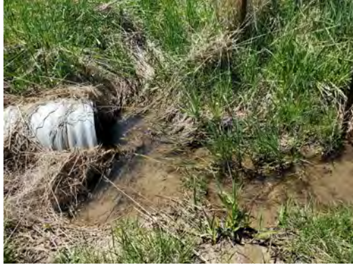
Photo 33: Location 12 – Culvert Inlet
