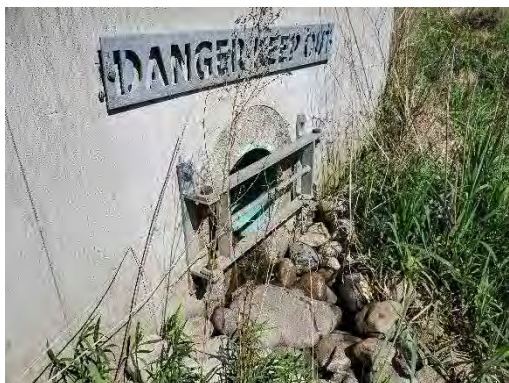
Photo 20: Location 8 – Outlet Upstream of Box Culvert
