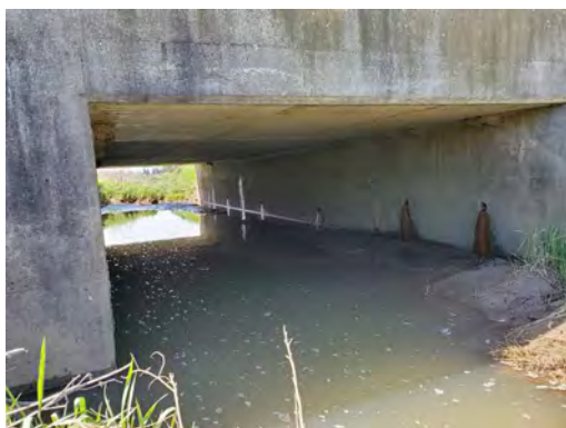
Photo 18: Location 8 – Box Culvert Upstream
