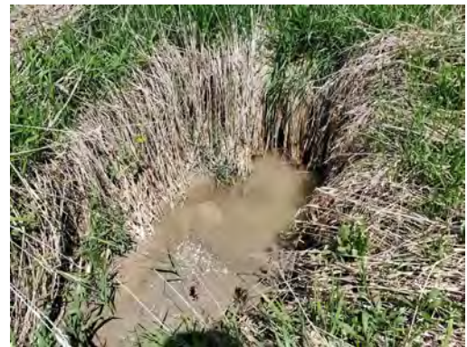
Photo 39: Location 14 – Culvert Outlet
