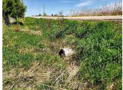
Photo 31: Location 11 – Culvert Inlet
