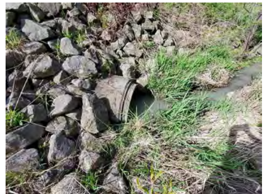
Photo 17: Location 7 – Culvert Outlet
