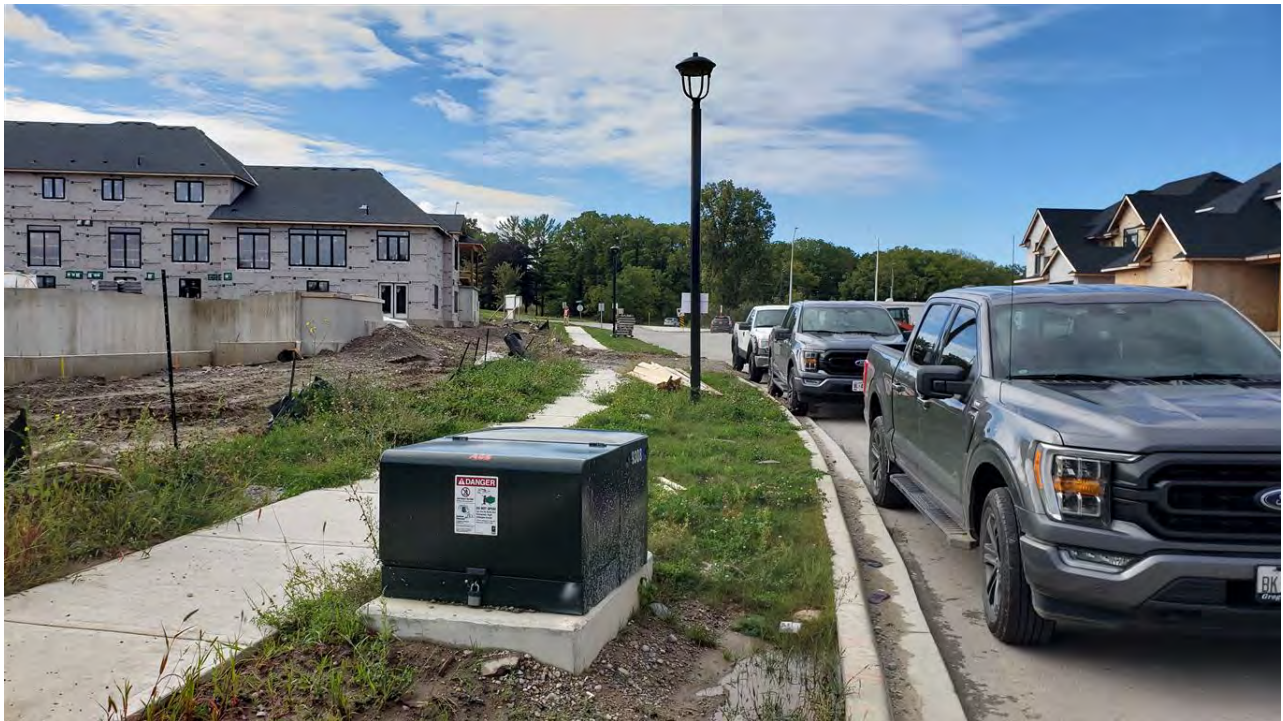
Image 15: A representative example of the disturbed Kains Road ROW; facing south, September 24, 2021.
