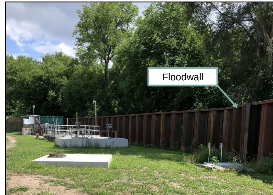
Floodwall at the Vauxhall Wastewater Treatment Plant (City of London)
