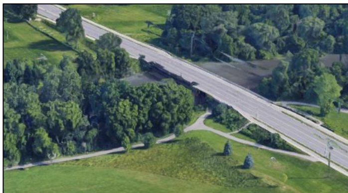
Adelaide Street Bridge (Image Source: Google Earth)
