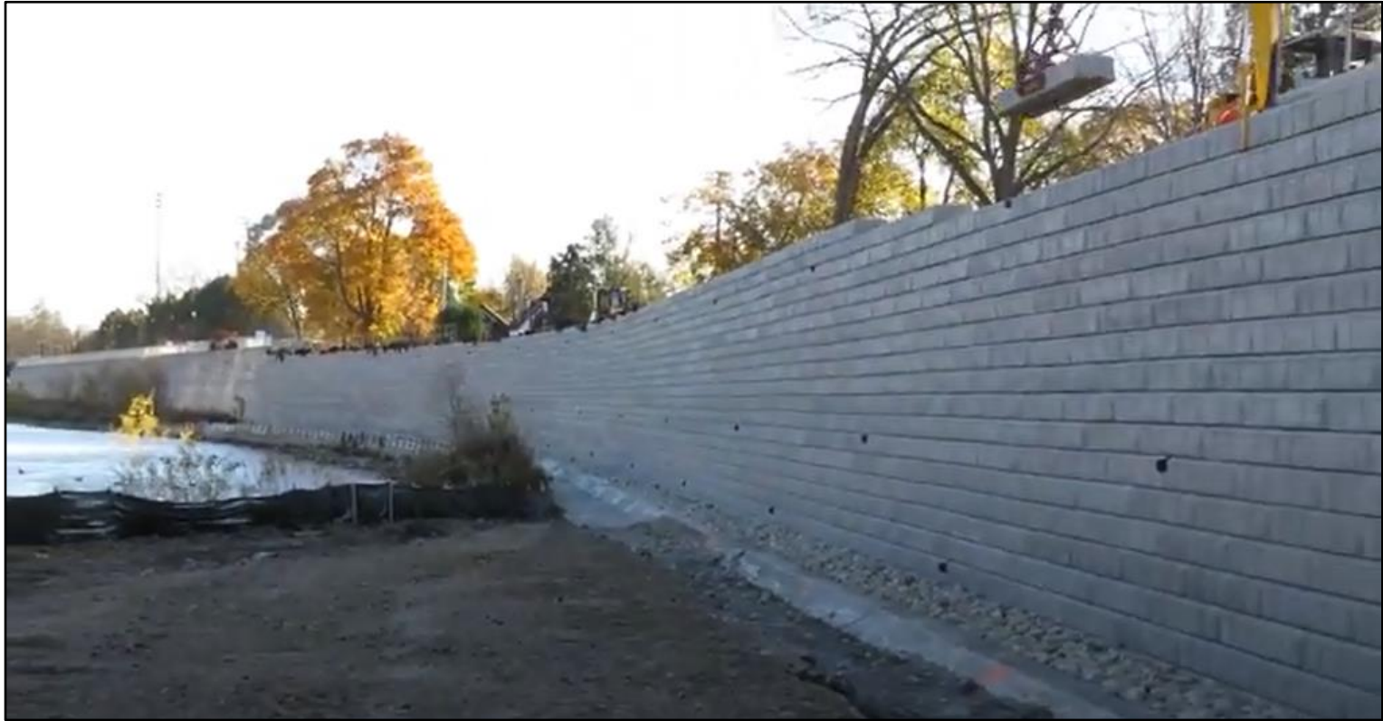
Construction of the West London Dyke (Image source: Upper Thames River Conservation Authority)
