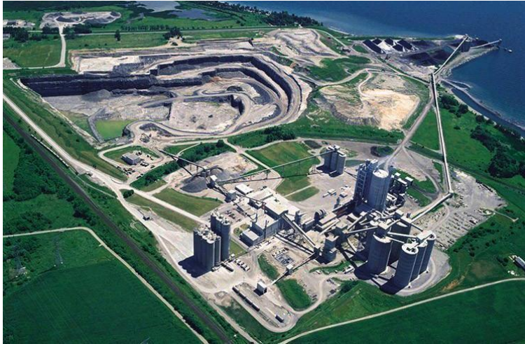
Figure 6. St. Mary's Cement facility in Bowmanville, ON that incorporates solids from the Duffin Creek Water Pollution Control Plant in their cement products. (Courtesy: http://www.stmaryscement.com/Pages/Media%20Centre/News/Cementing-the-future.aspx )
