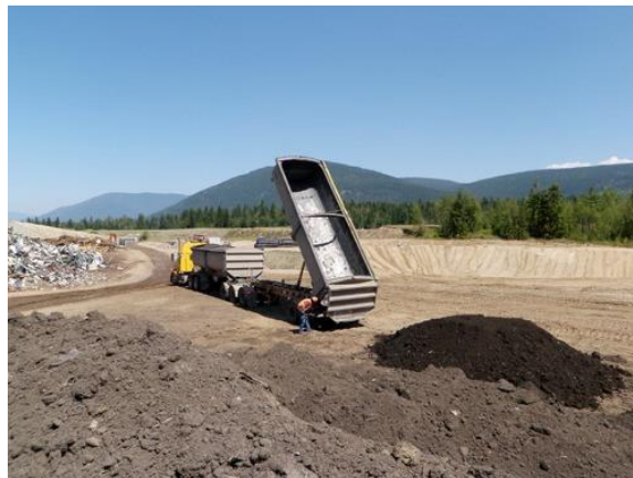
Figure 5. A truck unloading biosolids to a landfill in Vancouver (Courtesy: https://www.bcclocalnews.com/news/tnrd-utilizing-biosolids-to-close-landfills-in-region/ )
