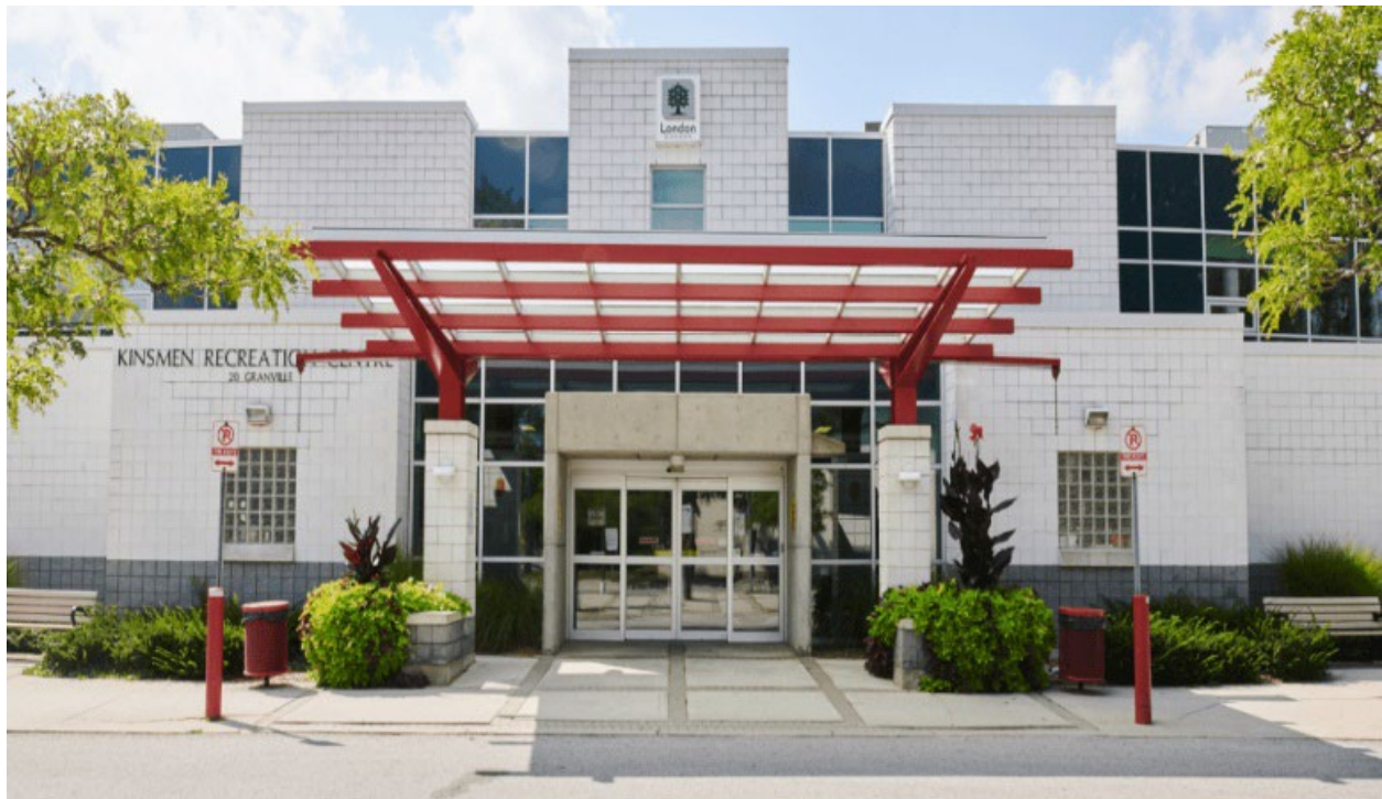
Figure 10 Kinsmen Arena Building
