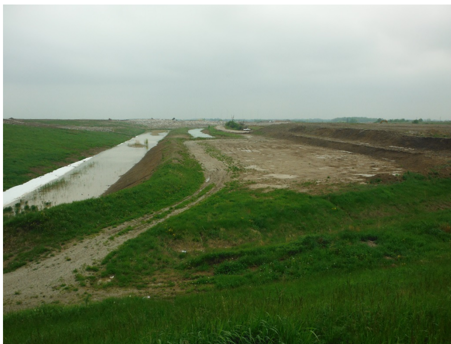
Image 3: Cells 9 and 10; Landfill construction along eastern boundary of Cells 9 and 10; facing south, May 22, 2018 (Map 8A).
