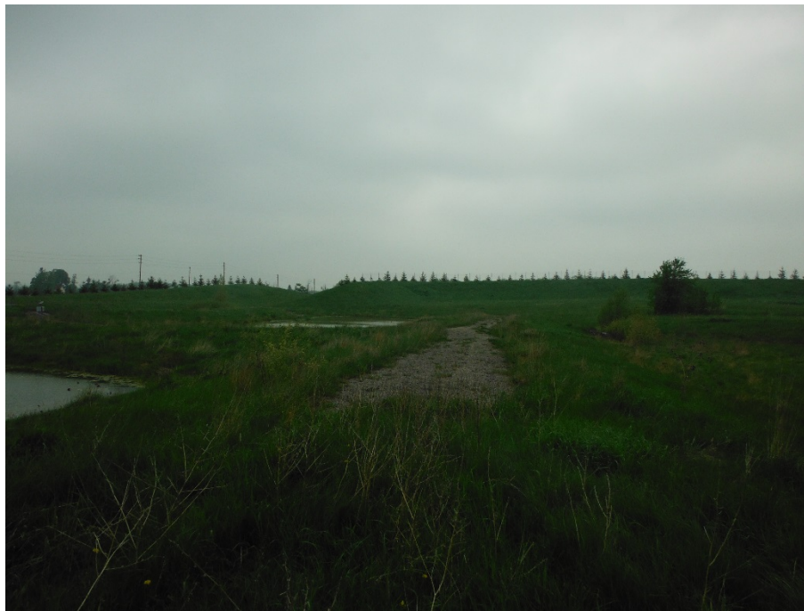
Image 21: Cells 9 and 10; Gravel access road and stormwater ponds; facing northwest, May 22, 2018 (Map 8A).
