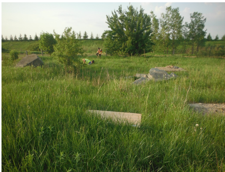
Image 23: Stockpile Area; Concrete footings; facing southeast, May 29, 2018.
