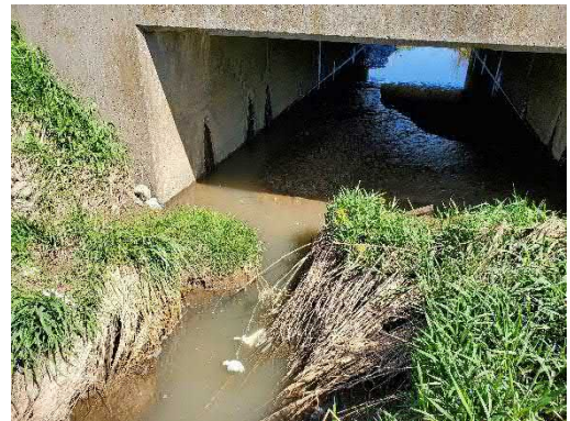
Photo 19: Location 8 – Box Culvert Downstream
