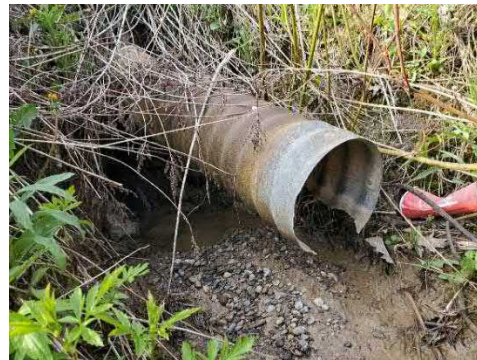
Photo 2: Location 1 – Culvert Outlet
