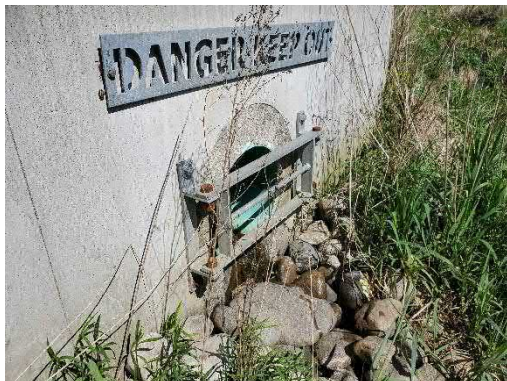
Photo 20: Location 8 – Outlet Upstream of Box Culvert
