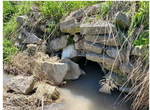
Photo 36: Location 13 – Culvert Inlet
