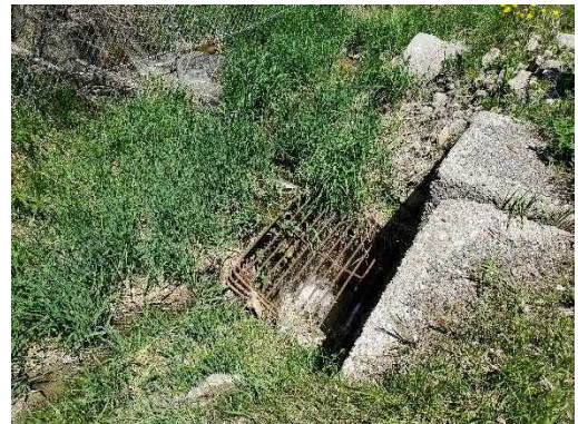
Photo 25: Location 9 – Grate Inlet near Culvert
