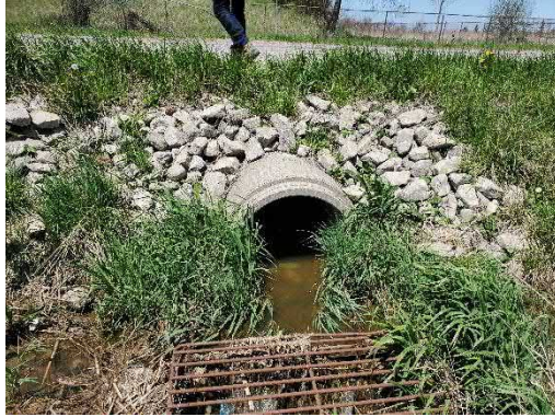
Photo 26: Location 9 – Culvert Outlet
