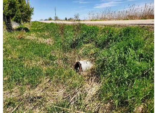
Photo 31: Location 11 – Culvert Inlet
