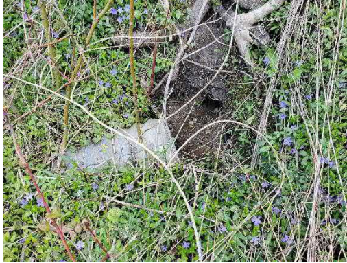
Photo 14: Location 6 – Culvert Inlet
