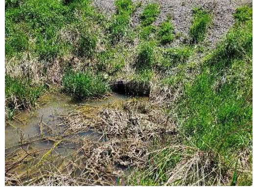
Photo 28: Location 10 – Culvert Inlet
