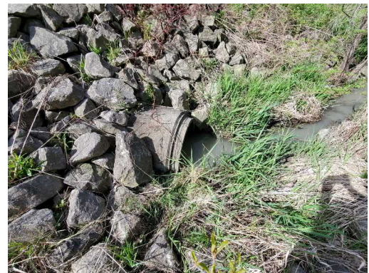
Photo 17: Location 7 – Culvert Outlet
