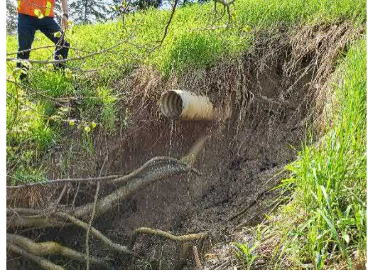
Photo 15: Location 6 – Culvert Outlet
