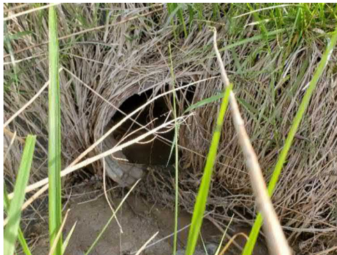
Photo 1: Location 1 – Culvert Inlet
