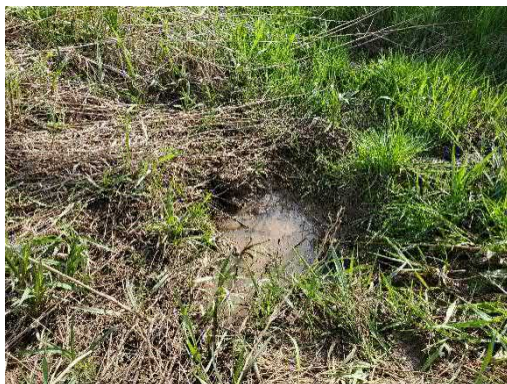
Photo 9: Location 4 – Culvert Inlet
