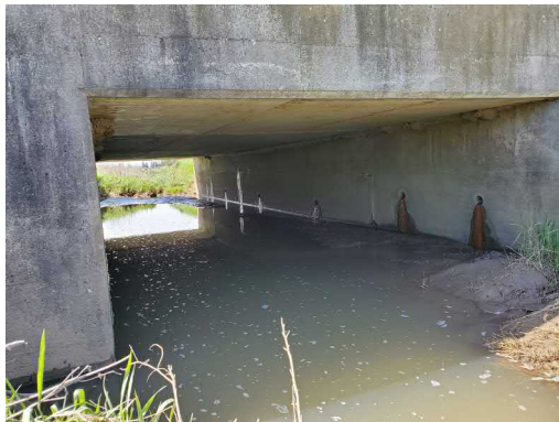
Photo 18: Location 8 – Box Culvert Upstream
