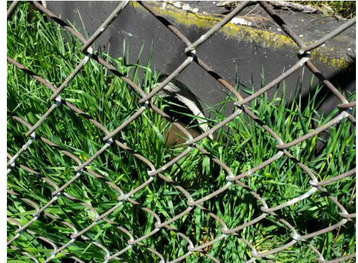
Photo 23: Location 9 – Pipe Outlet Upstream of Culvert
