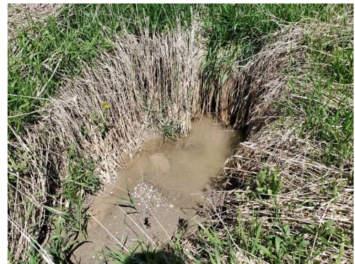
Photo 39: Location 14 – Culvert Outlet
