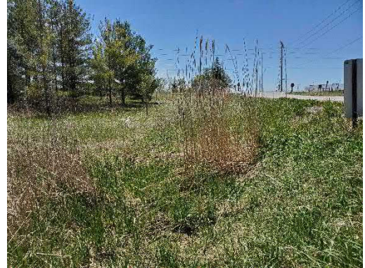
Photo 34: Location 12 – Culvert Outlet
