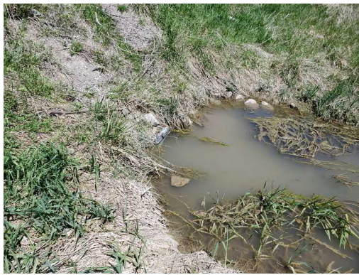
Photo 29: Location 10 – Culvert Outlet
