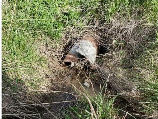
Photo 3: Location 2 – Culvert Inlet
