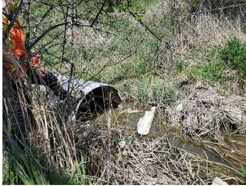
Photo 27: Location 10 – Outlet Pipe from Landfill
