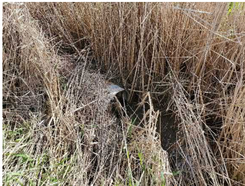
Photo 12: Location 5 – Culvert Inlet
