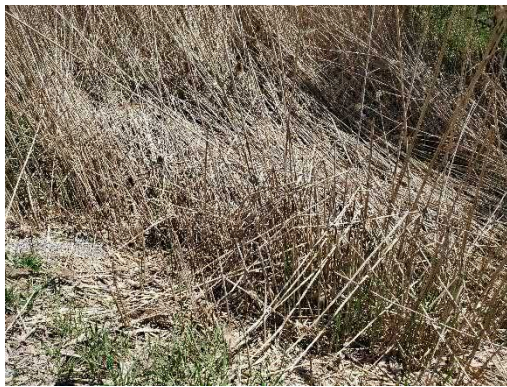
Photo 32: Location 11 – Culvert Outlet
