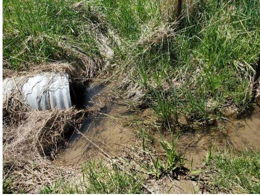
Photo 33: Location 12 – Culvert Inlet
