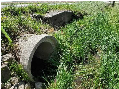
Photo 24: Location 9 – Culvert Inlet
