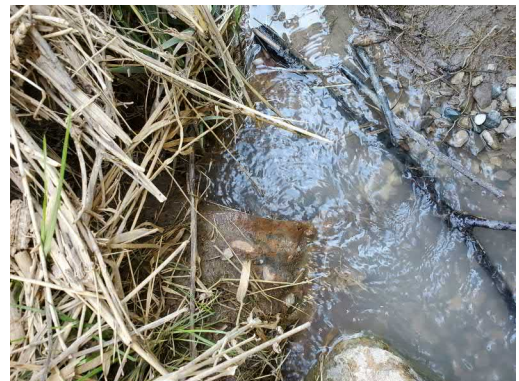
Photo 21: Location 8 – Outlet Upstream of Box Culvert
