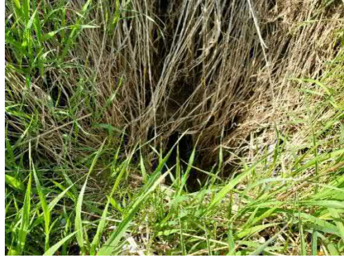
Photo 8: Location 3 – Culvert Outlet
