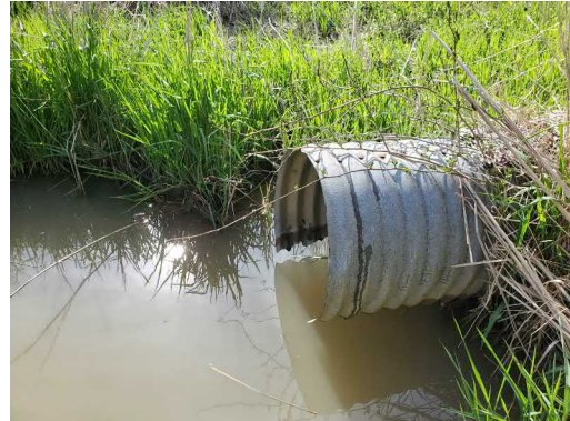
Photo 13: Location 5 – Culvert Outlet
