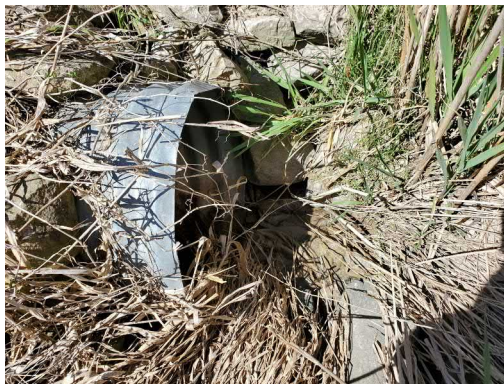
Photo 38: Location 14 – Culvert Inlet
