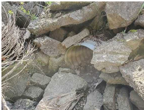
Photo 4: Location 2 – Culvert Outlet
