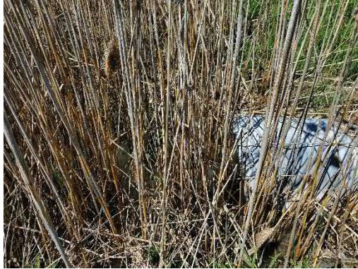
Photo 37: Location 13 – Culvert Outlet
