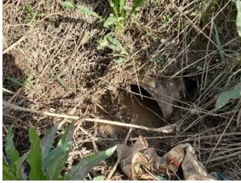
Photo 6: Location 3 – Culvert Inlet
