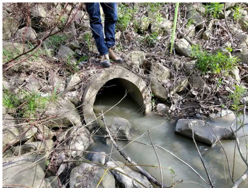
Photo 16: Location 7 – Culvert Inlet
