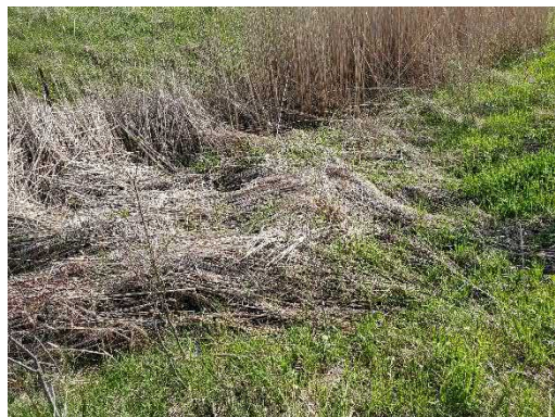
Photo 10: Location 4 – Culvert Outlet
