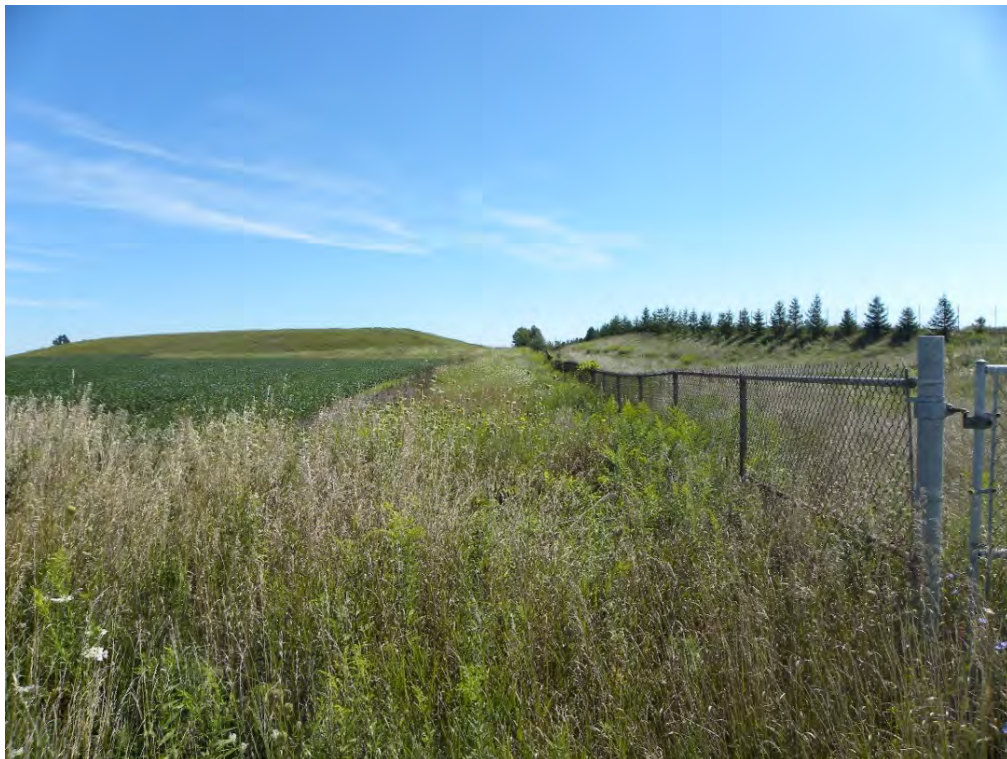
Figure 9: North Berm of the Existing W12A Landfill as Viewed from White Oak Road, Facing East
