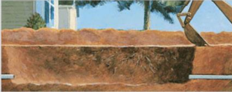
OPEN CUT EXCAVATION
