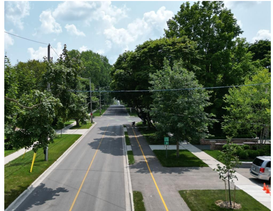
Existing two-way cycle track in the west boulevard on William Street looking southerly from Harrison Crescent
