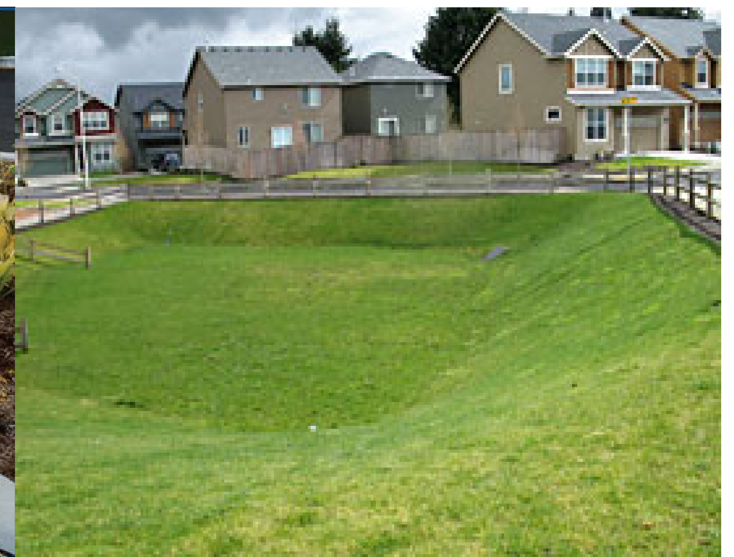
Dry SWM Facility
