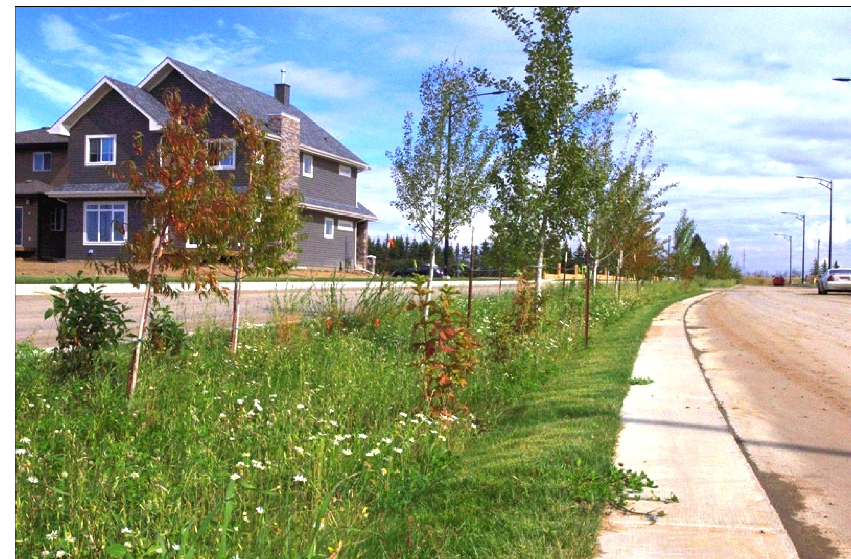
Example of a Low Impact Development feature (Bioswale)
