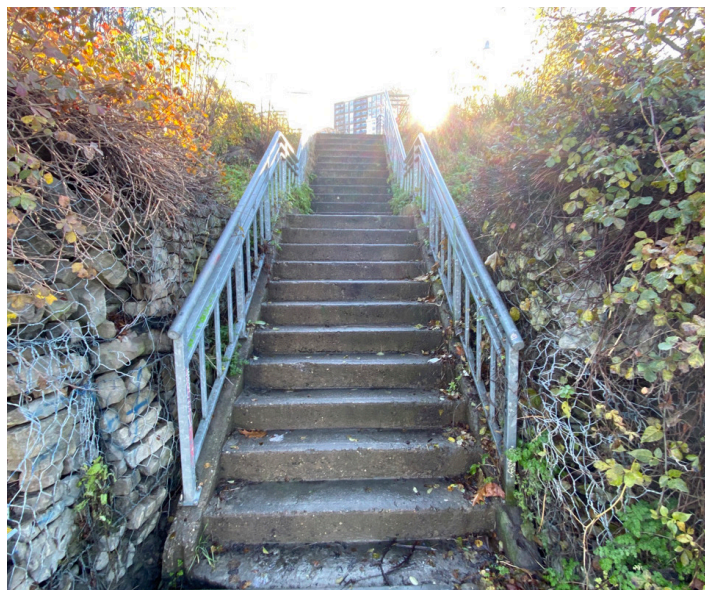
Figure 61: Existing Stairs Leading to Dock
