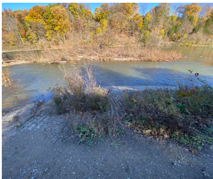
Figure 1: View of Shore Access- Concrete Mats
