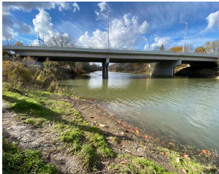
Figure 40: Existing Shore Access- Easy Access
