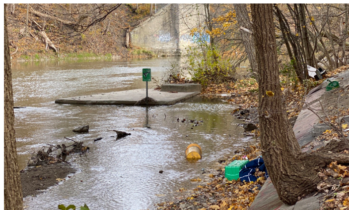
Figure 46: Existing Launch East of Weir- Cannot Access due to Water Levels; Lots of Garbage in this Area
