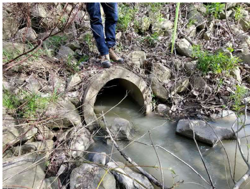
Photo 16: Location 7 – Culvert Inlet
