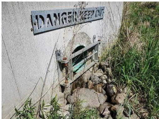
Photo 20: Location 8 – Outlet Upstream of Box Culvert
