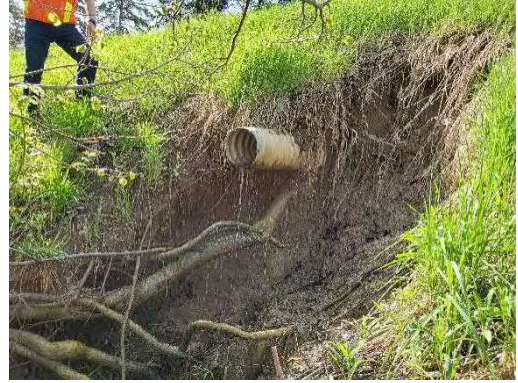
Photo 15: Location 6 – Culvert Outlet
