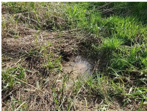
Photo 9: Location 4 – Culvert Inlet
