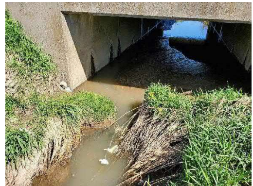
Photo 19: Location 8 – Box Culvert Downstream
