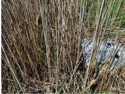
Photo 37: Location 13 – Culvert Outlet
