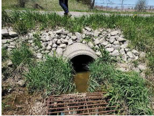
Photo 26: Location 9 – Culvert Outlet
