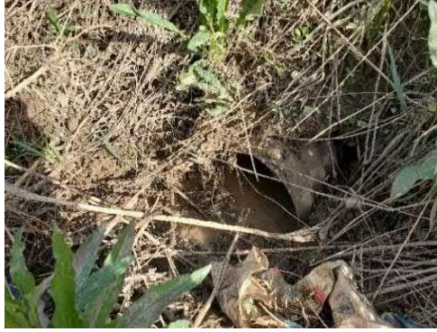
Photo 6: Location 3 – Culvert Inlet
