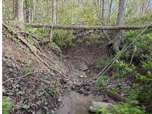
Photo 5: Location 2 – Downstream Channel
