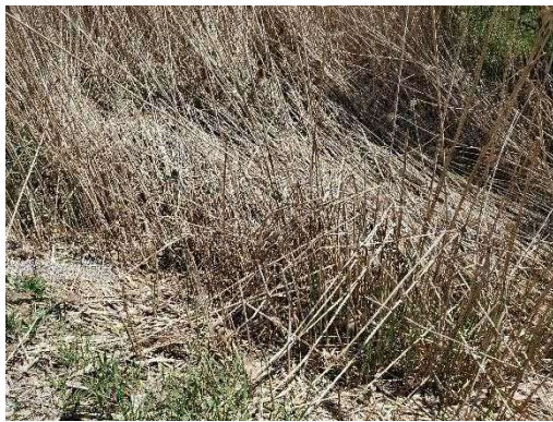
Photo 32: Location 11 – Culvert Outlet
