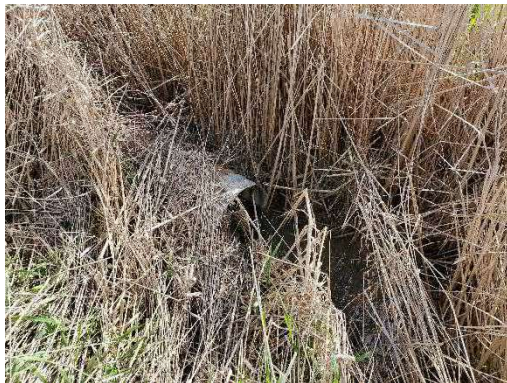
Photo 12: Location 5 – Culvert Inlet
