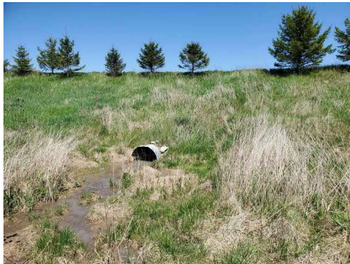
Photo 35: Location 13 – Outlet Pipe From Pond 1
