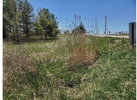
Photo 34: Location 12 – Culvert Outlet
