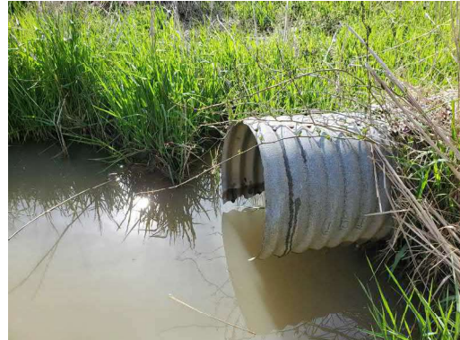
Photo 13: Location 5 – Culvert Outlet
