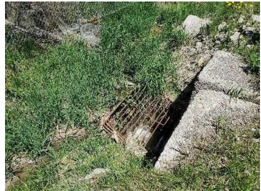
Photo 25: Location 9 – Grate Inlet near Culvert
