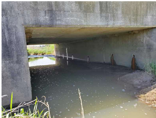
Photo 18: Location 8 – Box Culvert Upstream
