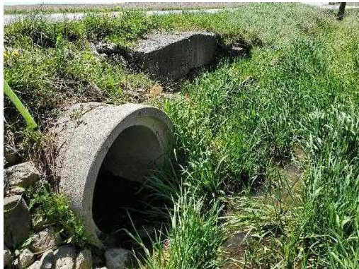
Photo 24: Location 9 – Culvert Inlet
