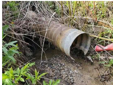
Photo 2: Location 1 – Culvert Outlet
