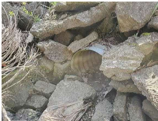
Photo 4: Location 2 – Culvert Outlet
