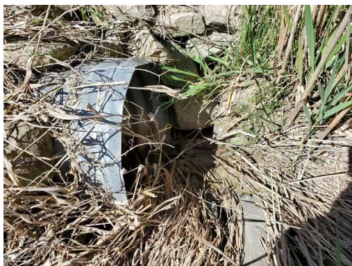
Photo 38: Location 14 – Culvert Inlet
