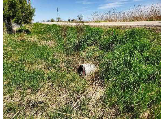
Photo 31: Location 11 – Culvert Inlet
