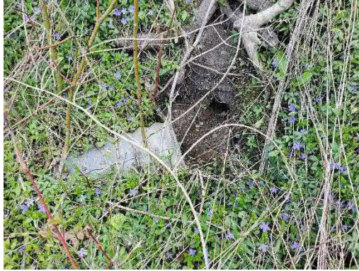
Photo 14: Location 6 – Culvert Inlet
