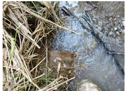
Photo 21: Location 8 – Outlet Upstream of Box Culvert
