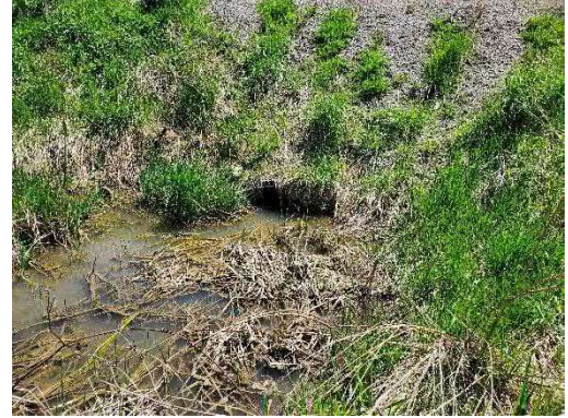
Photo 28: Location 10 – Culvert Inlet
