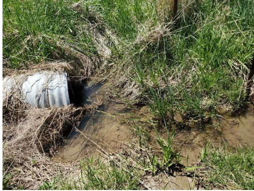
Photo 33: Location 12 – Culvert Inlet
