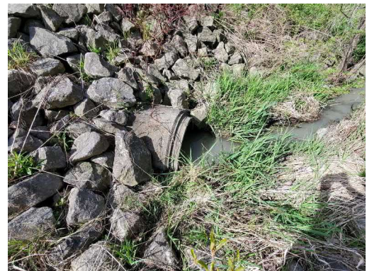
Photo 17: Location 7 – Culvert Outlet
