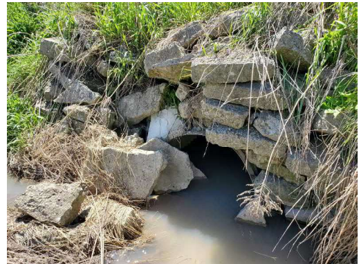
Photo 36: Location 13 – Culvert Inlet
