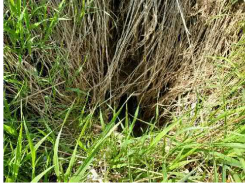
Photo 8: Location 3 – Culvert Outlet
