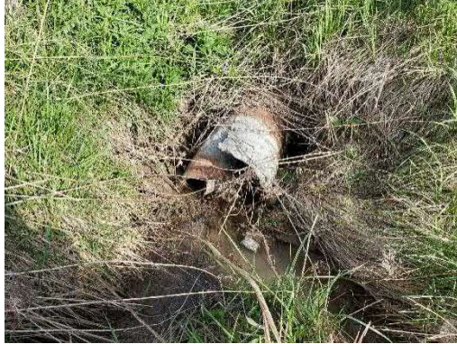
Photo 3: Location 2 – Culvert Inlet
