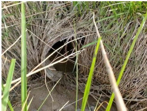
Photo 1: Location 1 – Culvert Inlet
