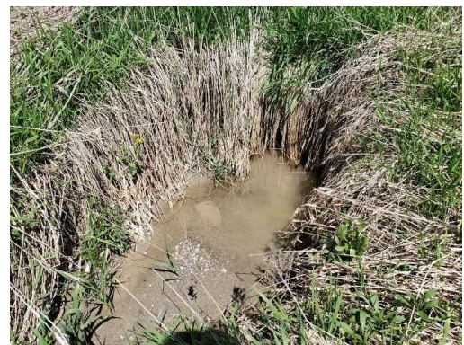
Photo 39: Location 14 – Culvert Outlet
