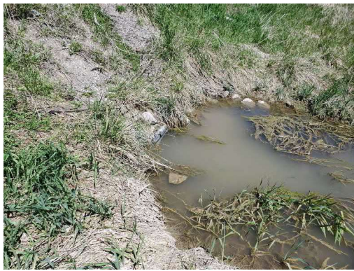
Photo 29: Location 10 – Culvert Outlet
