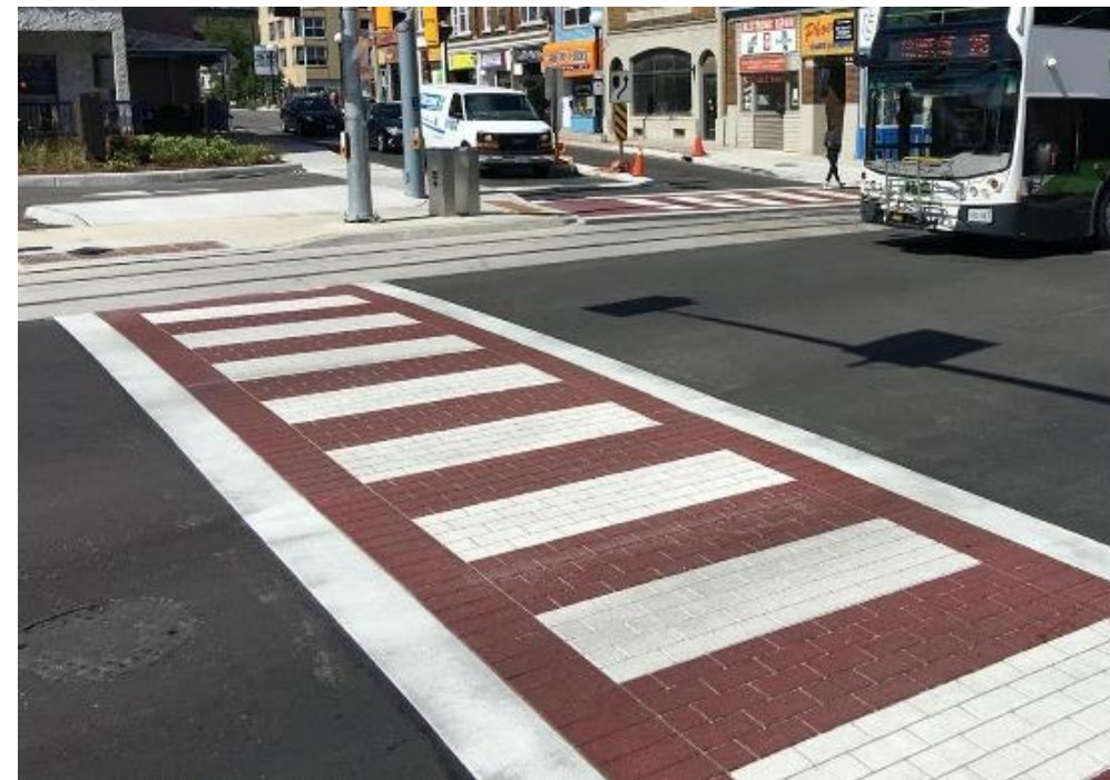
Enhanced pedestrian crossings at station stops
