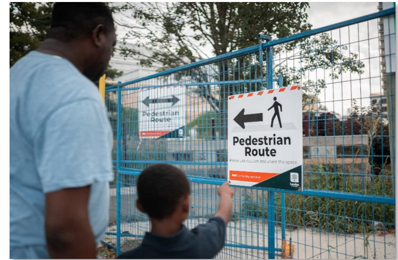
Wayfinding signs to help communicate construction plans, detours and timelines
