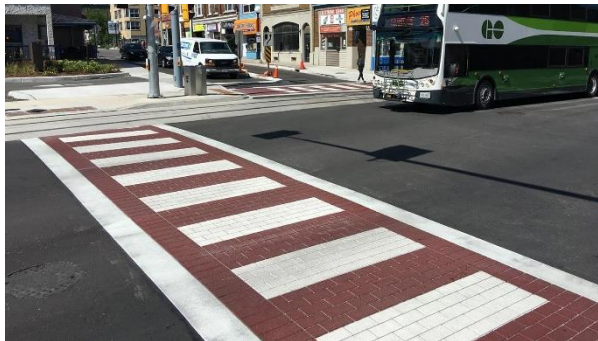
Enhanced pedestrian crossings at station stops
